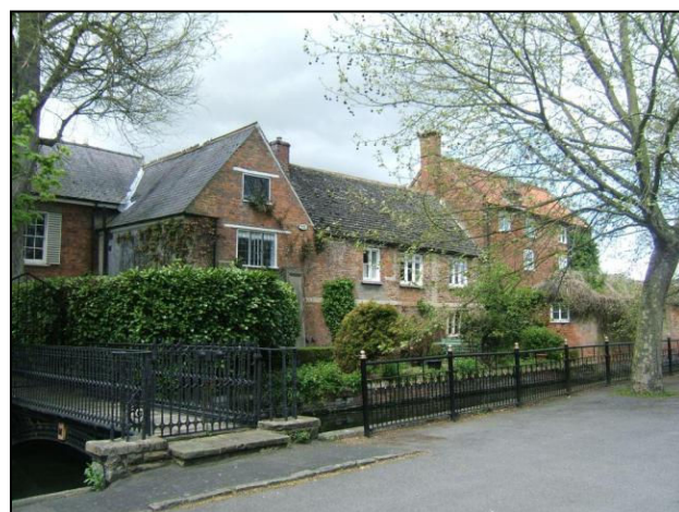
Fig.17 The Cedars (grade II listed) provides an attractive focus to Church Walk; to the left the footbridge which is also grade II listed.
